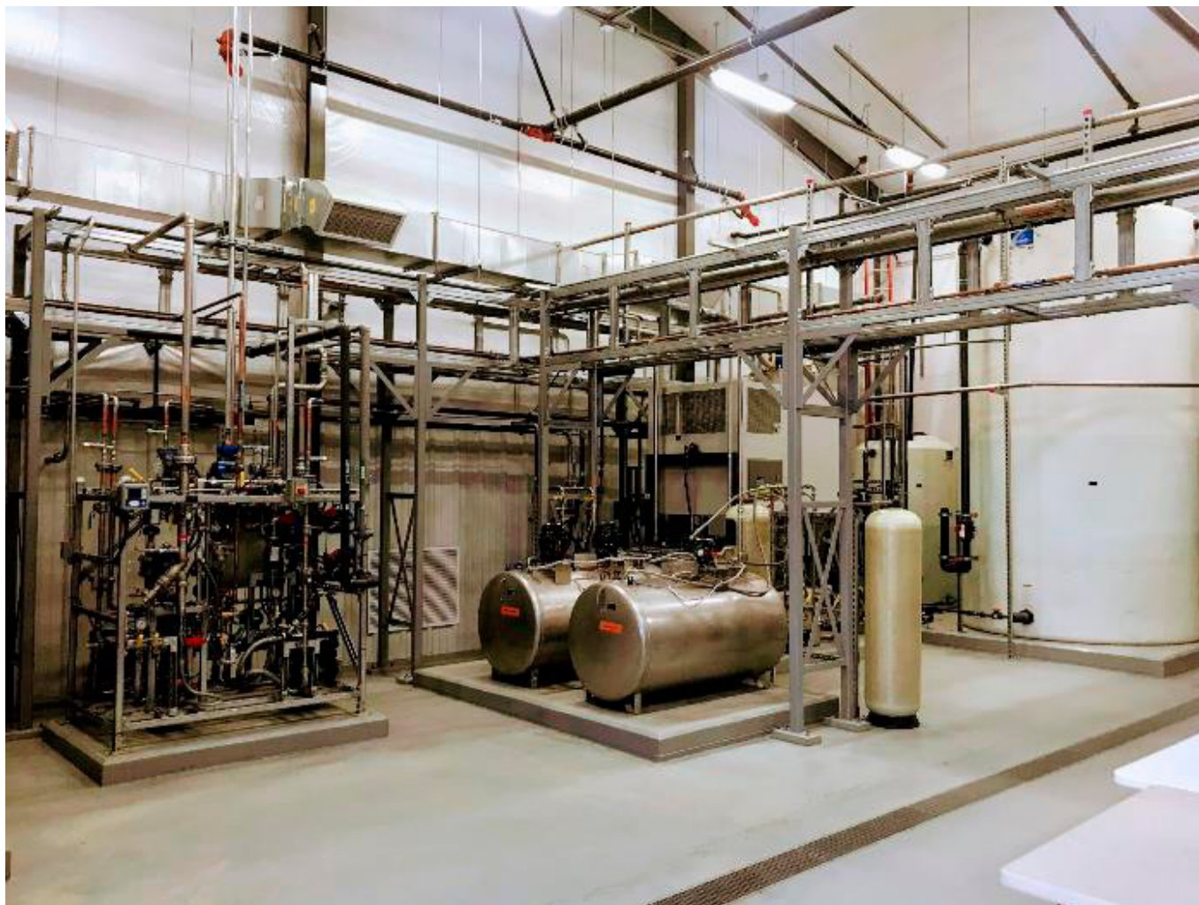
Figure 15-12. Resin regeneration system.
