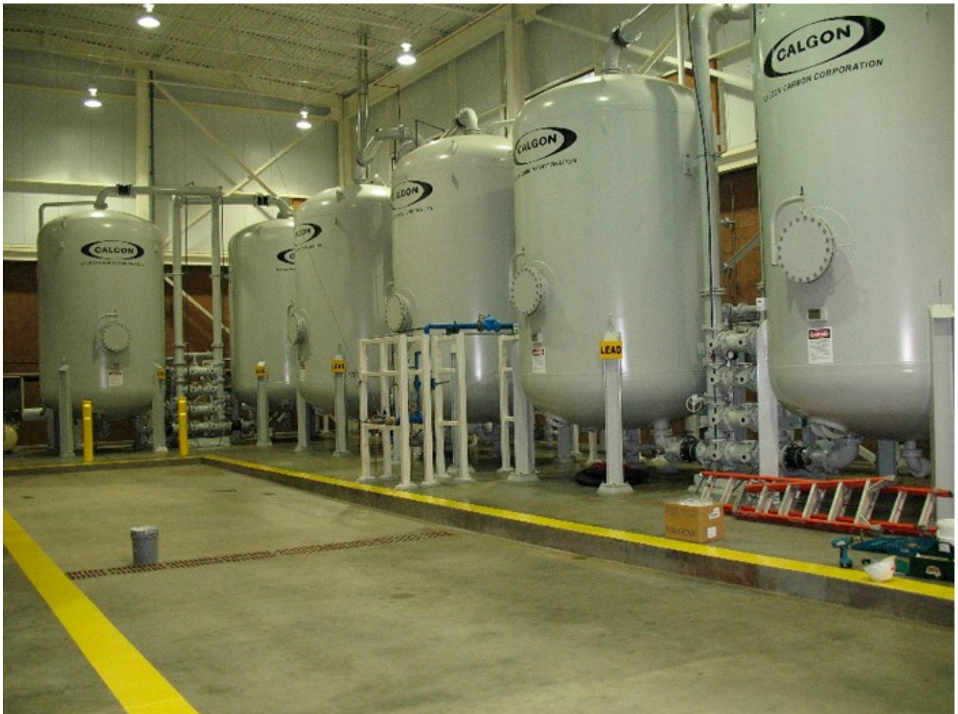
Figure 15-4. GAC treatment system, Oakdale, MN.
