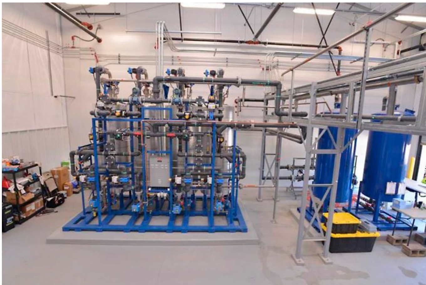
Figure 15-11. Regenerable and polish IX resin vessel skids.
